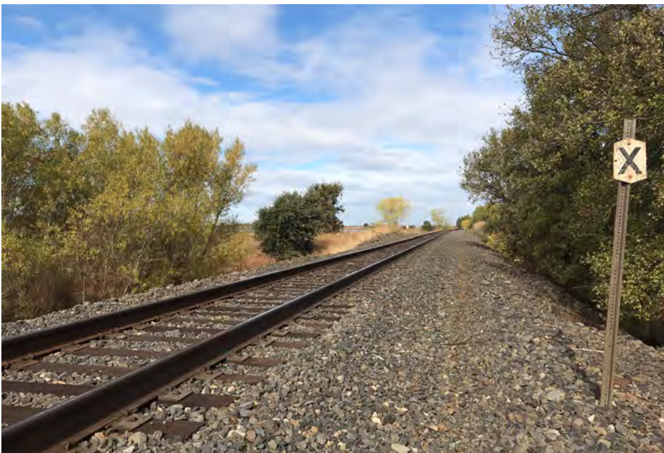
Photograph 12. South end of Segment 6, camera facing north, November 10, 2017
