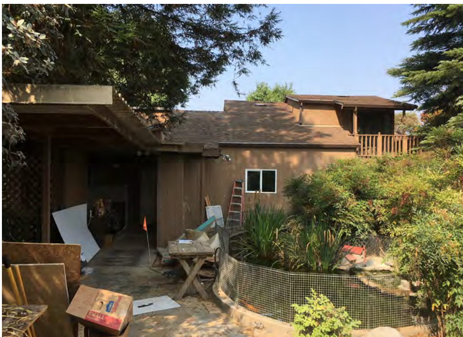
Photograph 3. East side of Building 1, camera facing west, August 22, 2018
