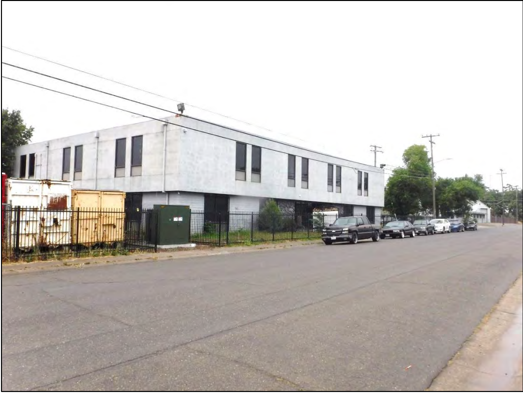
Photograph 5. Office Building (view northwest)
