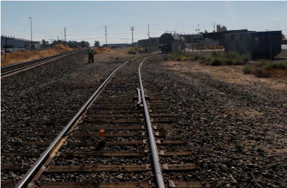
Photograph 2. Siding on west side of the Segment 1 of UPRR, north of W. Elkhorn Boulevard, camera facing southwest, October 27, 2017
