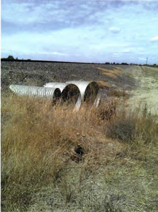
Pic. 200: Three culverts running under ballast, taken facing 323°.
