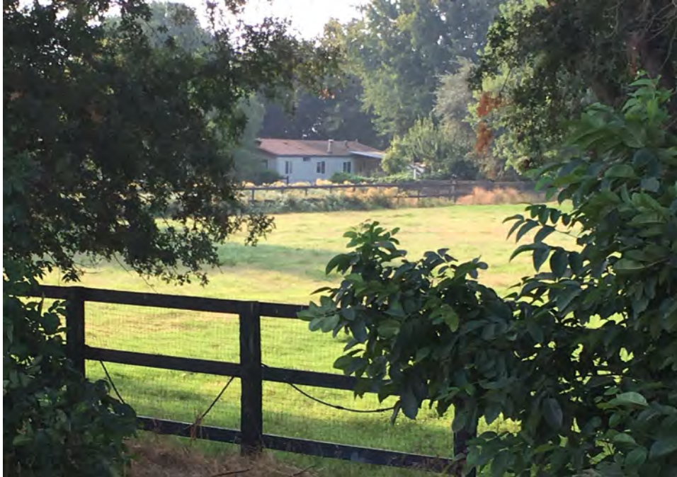
Photograph 3. North and west sides of Building 1, taken from Highway 12, camera facing southeast, August 22, 2018
