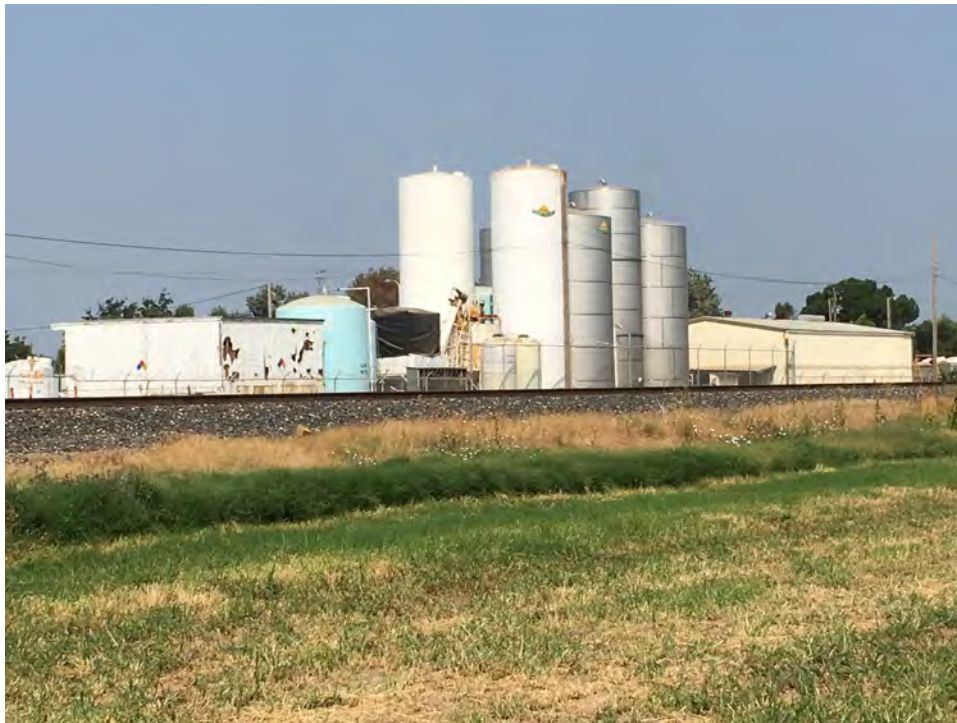
Photograph 6. South and east sides of flammable storage shed in foreground, tanks at center, and northern warehouse in background, camera facing northwest August 22, 2018
