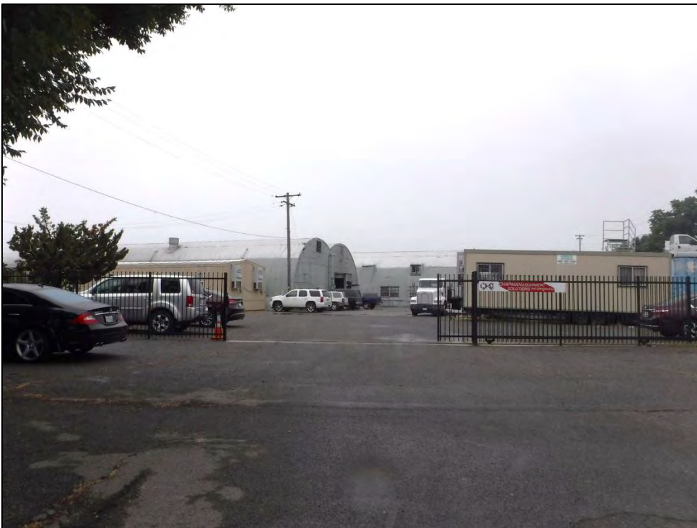
Photograph 2. East and Rear (North) Elevations of Quonset Huts (view west)
