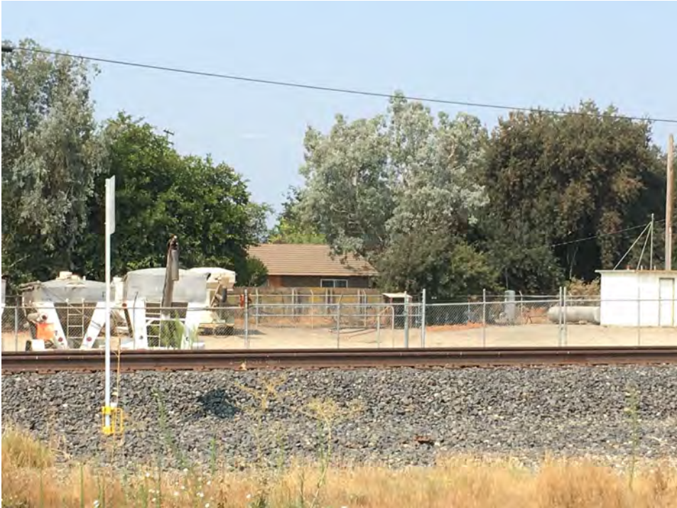
Photograph 2. East side of residence showing replacement windows and siding, railroad tracks in foreground, camera facing west, August 22, 2018
