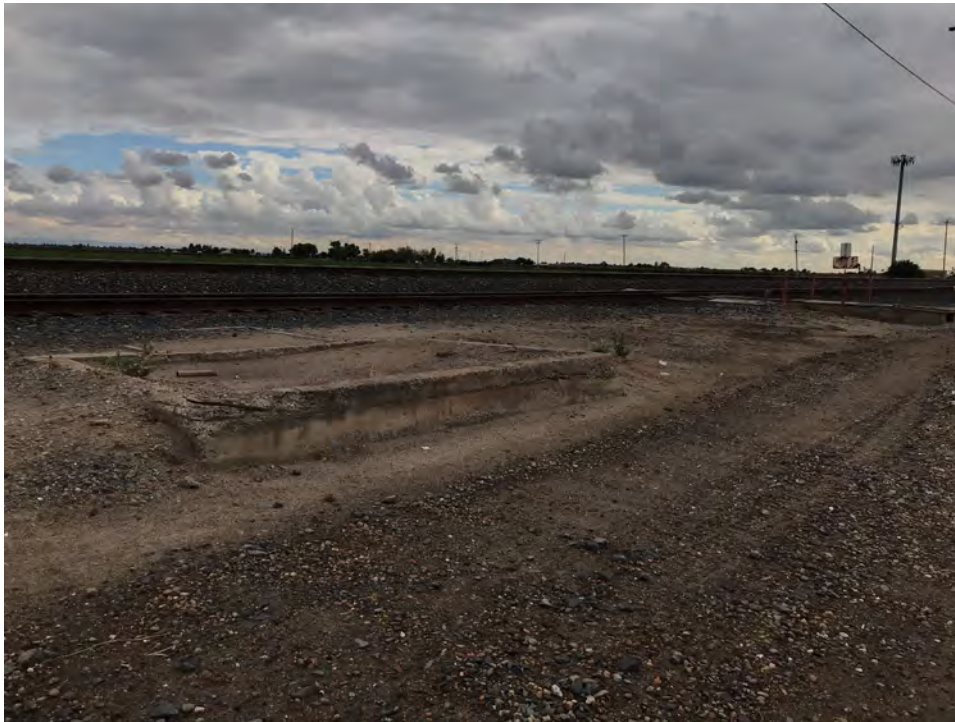
Photograph 5. Concrete foundations (on left) and concrete box vault with plywood cover, associated with the former dry hopper loading area (on right), both located in the railroad right-of-way. Camera facing southeast, November 9, 2017
