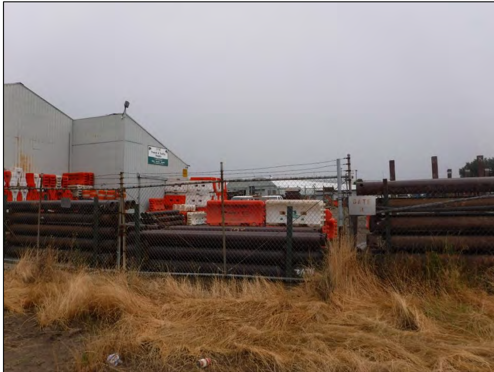
Photograph 4. Lean-To Addition on Northeast Corner of Warehouse (view north)
