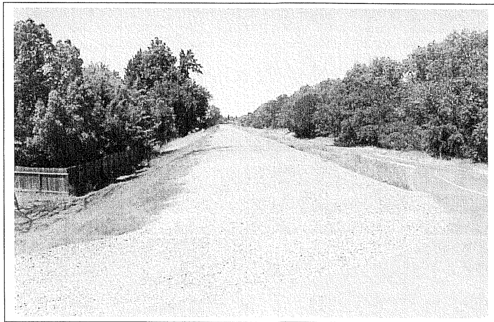
Photograph 3. REF 47-H, left bank levee
