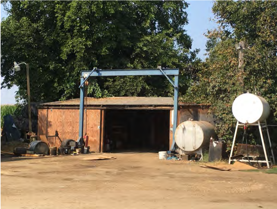
Photograph 4. East side of Building 2, camera facing southwest, August 22, 2018
