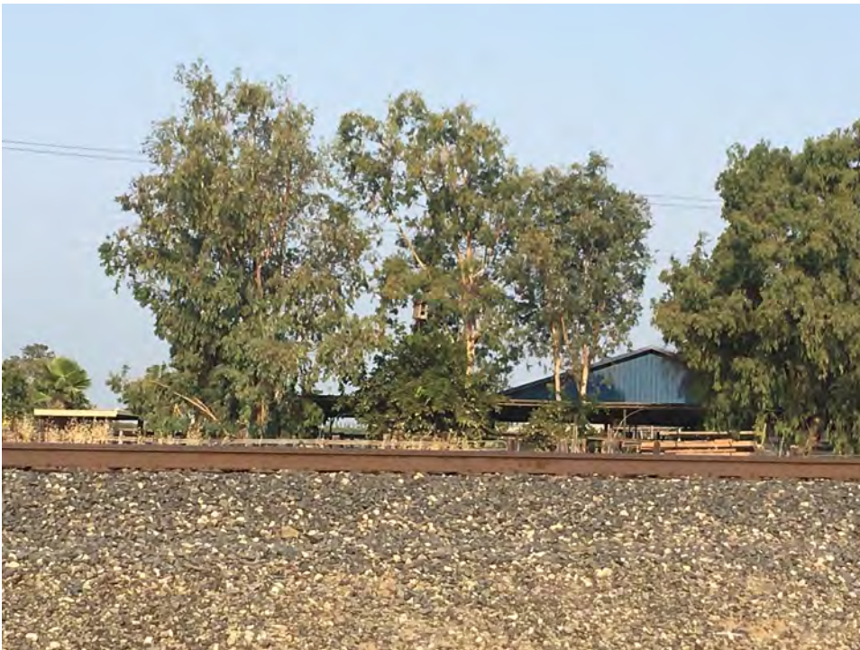
Photograph 8. East side of Building 8 (blue gable), Shelter 5 in center foreground (flat roof), and Shelter 6 on far left, facing west, August 22, 2018
