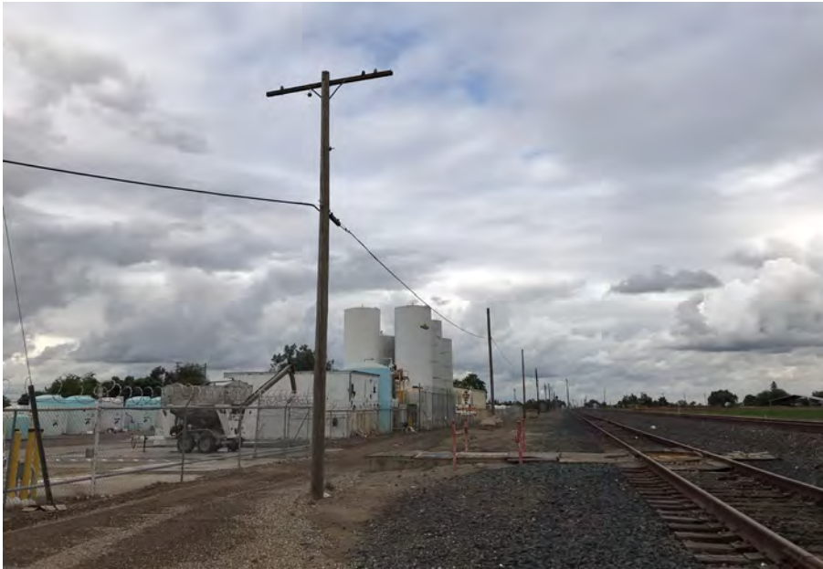
Photograph 5. Segment 2 of WPRR at Simplot Siding, camera facing northwest, November 9, 2017
