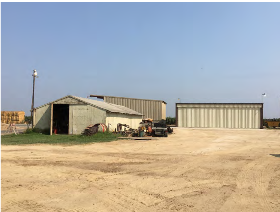
Photograph 13. From left to right: Building 11, Building 9, Building 10, camera facing northwest, August 22, 2018
