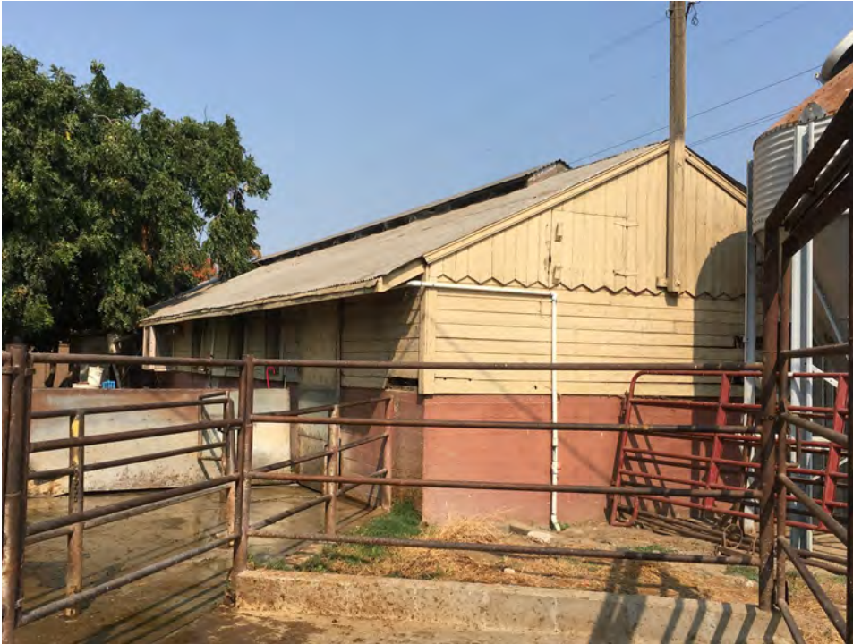
Photograph 6. South and east sides of Building 3, camera facing northwest, August 22, 2018
