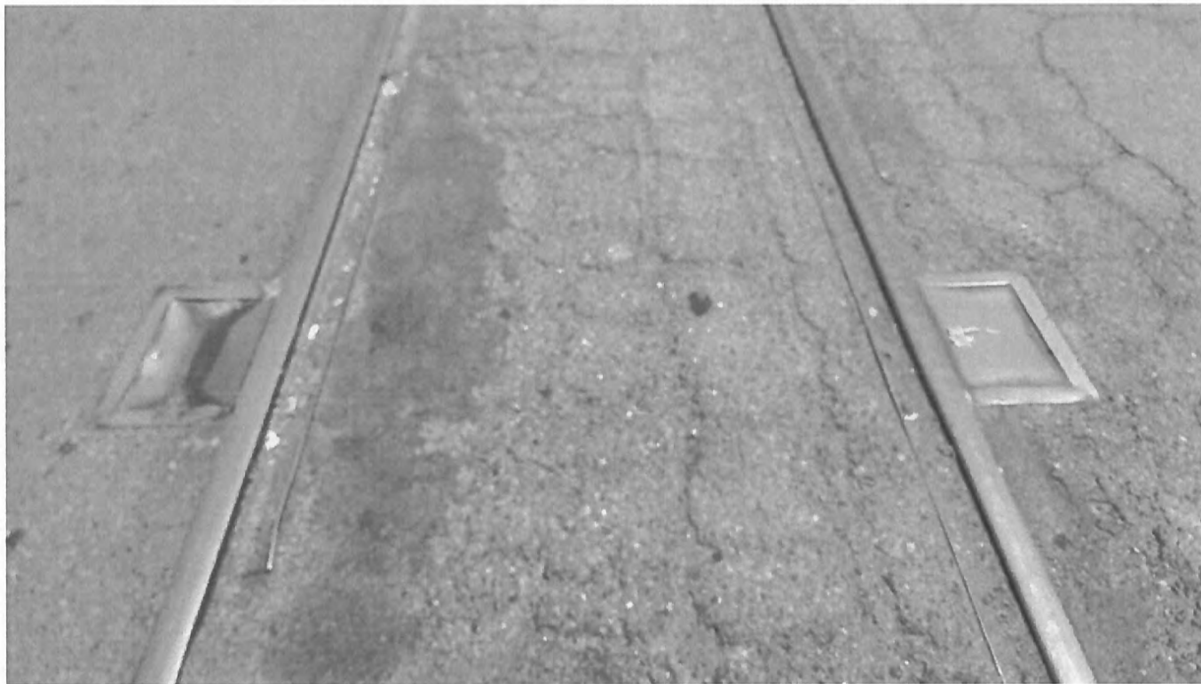
Siding feature, east of 14 th /R Street intersection, View east, 5-15-14, IMG#498
