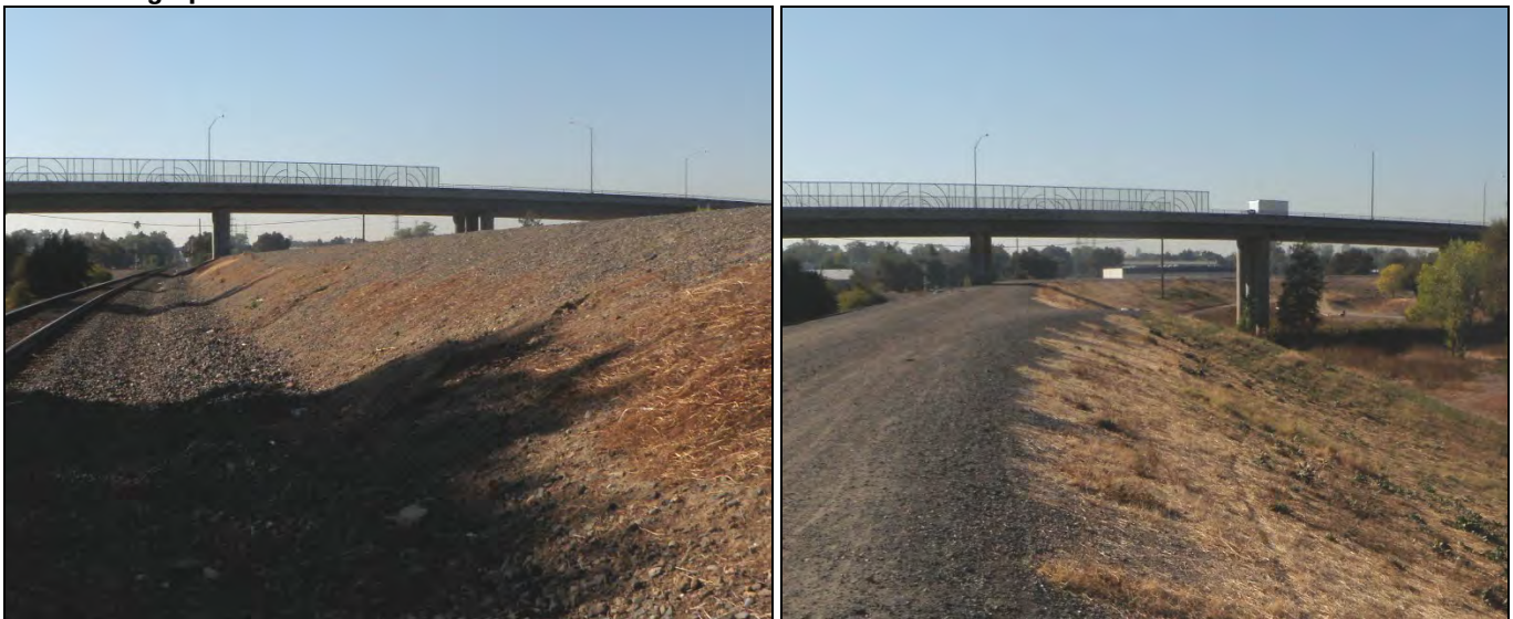
Photograph 1 (Left). UPRR track (left) on east side of levee with the Arden Way-Garden Highway Connector in background, October 27, 2017
