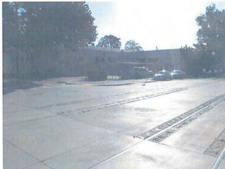
View Northeast down R Street from 13 th Street, 8-1-2013, DIG#327
