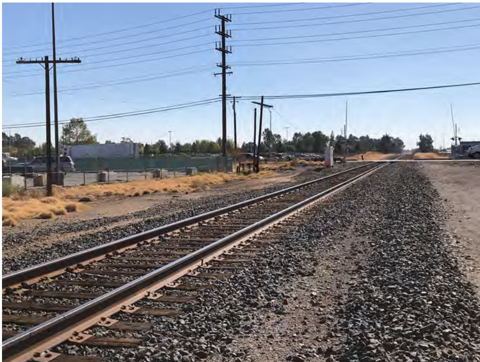
Photograph 2. South End of Segment of Telegraph Poles, with West Elkhorn Boulevard railroad crossing in background, camera facing southwest, October 26, 2017
