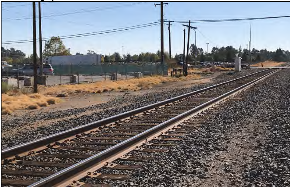
Photograph 1. Segment 1 of UPRR, north of W. Elkhorn Boulevard, camera facing southeast, October 27, 2017
