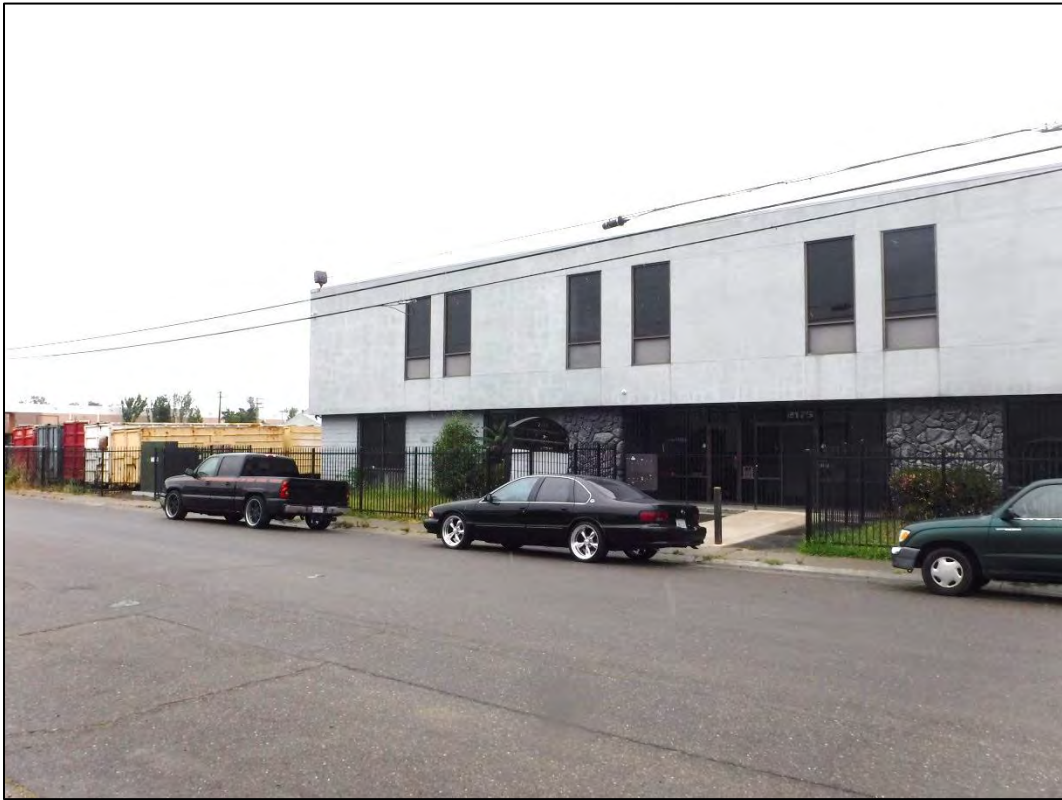
Photograph 6. Office Building (view southwest)
