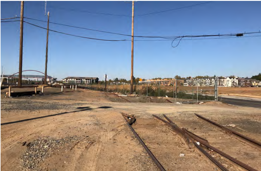
Photograph 9. Segment 4 showing entrance into layover yard from 10 th Avenue, just north of the Sutterville Road overpass, showing abandoned frog tracks, camera facing north, October 27, 2017
