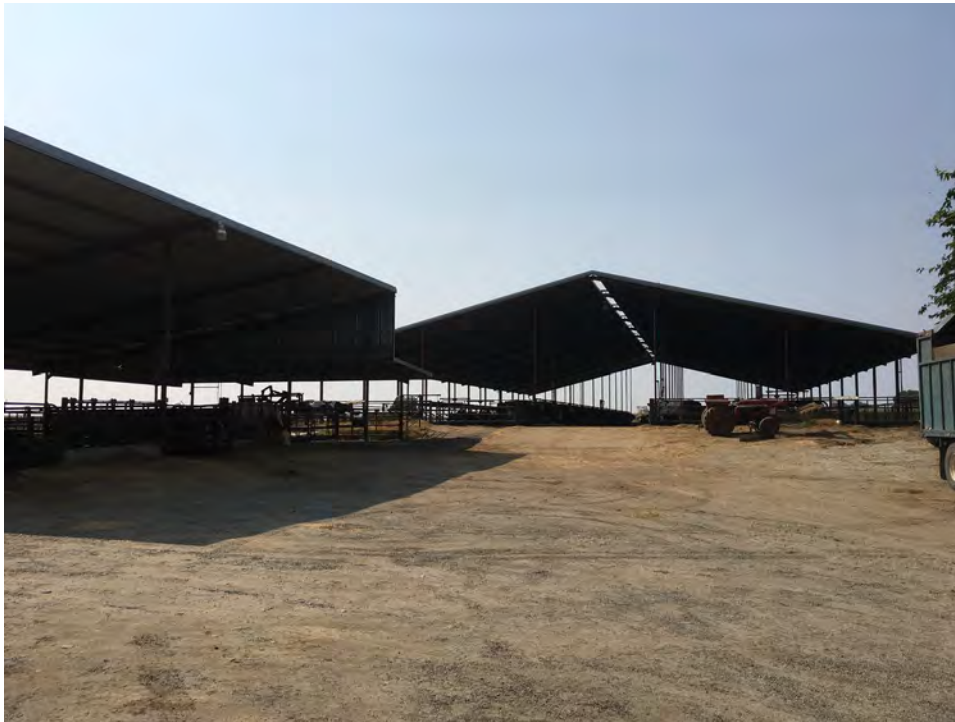
Photograph 10. Building 5 on left, Building 6 on right, camera facing south, August 22, 2018
