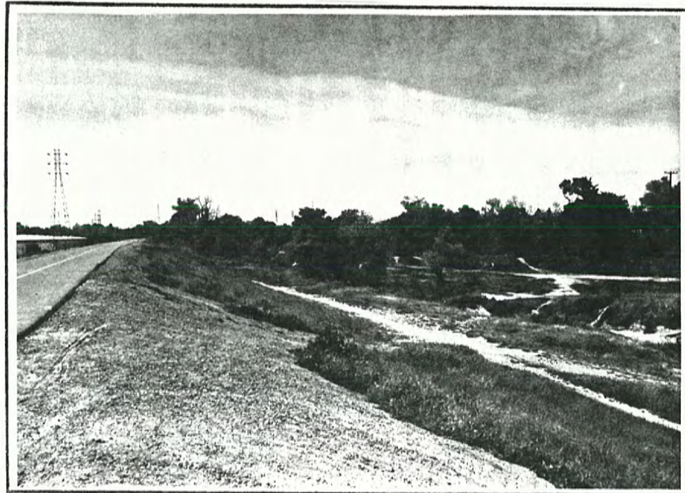
Canal floodplain from bicycle path, View to southwest.
