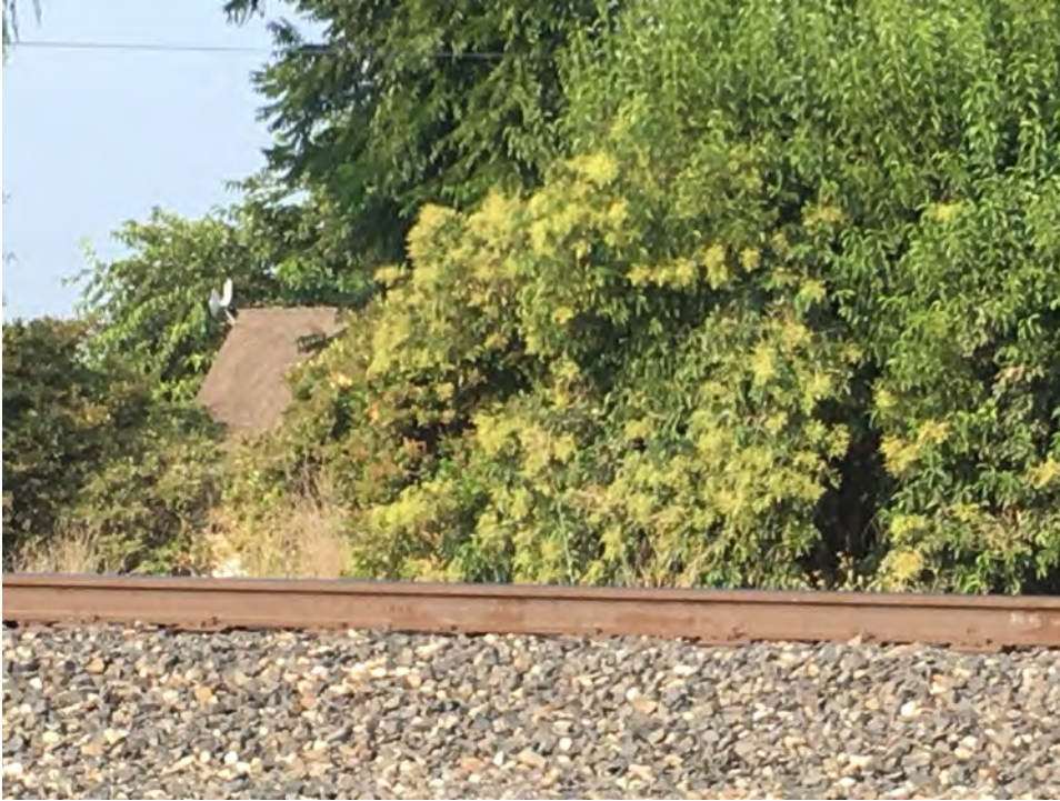
Photograph 5. South end of gable roof on Building 4, camera facing west, August 22, 2018
