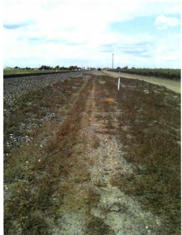
Pic. 204: RR 3 tiered ballast section with fiberoptic post, facing 341°.
