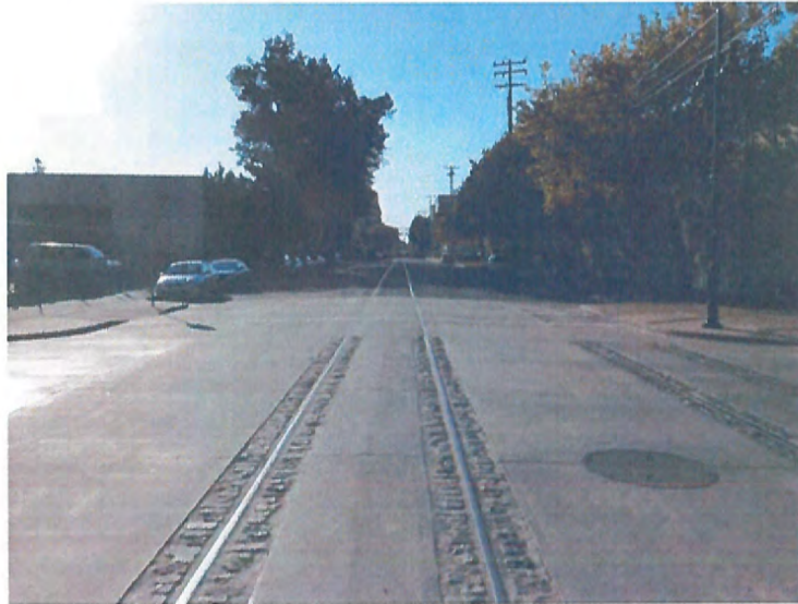
Main Track and Siding, View East down R Street from 13 th Street, 8-1-2013, DIG#326
