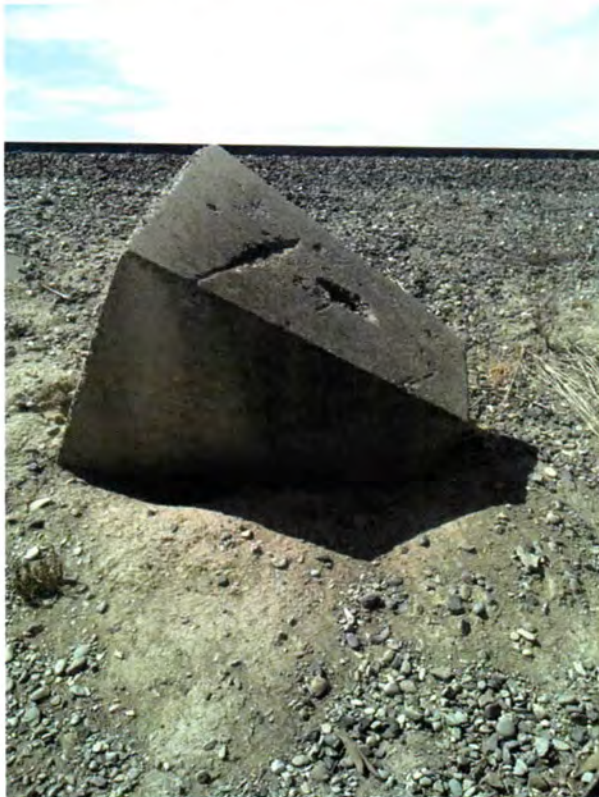
Pic. 203: Large cement block, taken facing 247°.
