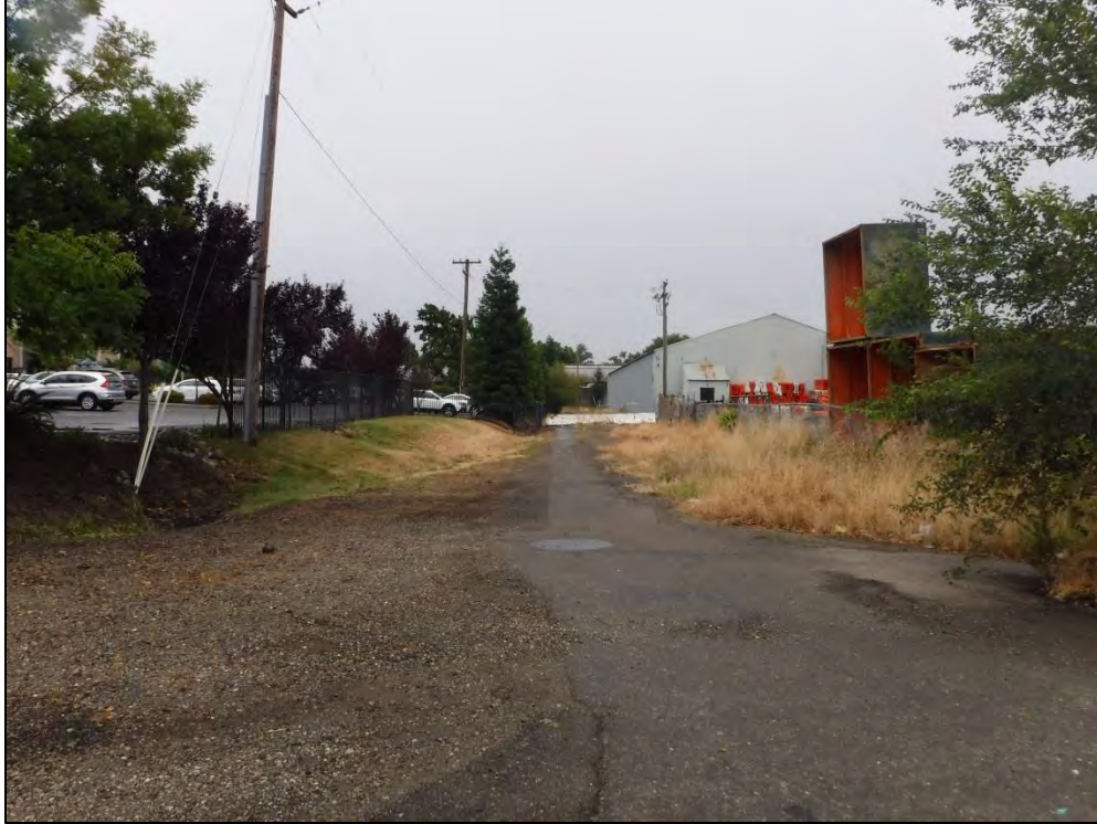
Photograph 3. South and East Elevations of Warehouse (view west)
